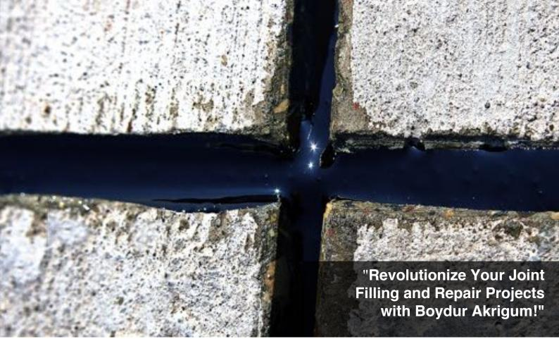
Let me introduce you to Boydur Akrigum, a professional-grade, methyl methacrylate (MMA) based, two-component, flexible repair and joint filling solution. It is designed for both indoor and outdoor applications, offering exceptional versatility and performance.
